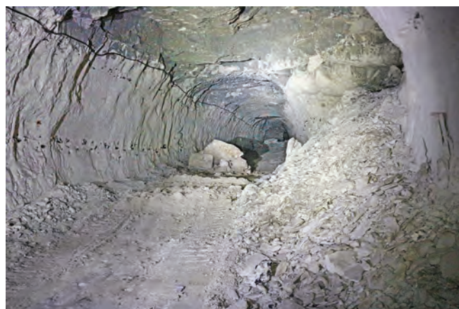
A soot blackened unfinished drift reveals layers of flint within the chalk. Photo Bob Clary
